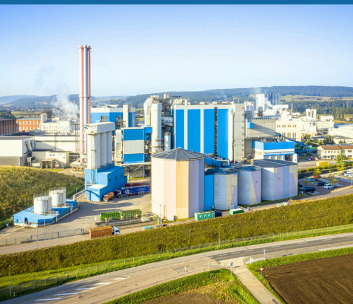
Photo: the Schwandorf WtE plant in Germany. ©Silke Reents
